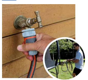
Connect a hose to an outdoor water source, and run it to the base of the trampoline, ready to be connected. Choose one of the net poles as your desired connection point. The misting tube will run down the length of this net pole.
